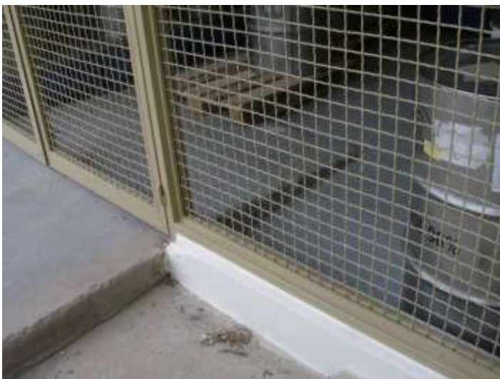
Secondary containment of the same area.
