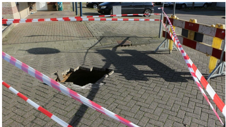
Insufficient barricading during paving maintenance works.
