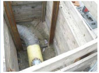
Excavation/ trenching rigid protection from wall collapse at a maintenance worksite in Berlin.
