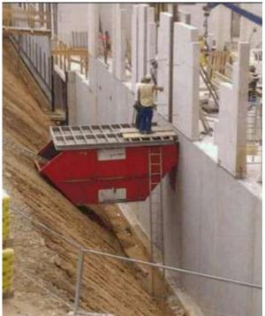
Poor improvisation for providing a working/ access platform in a worksite; the access ladder is also a substandard hazardous practice.
