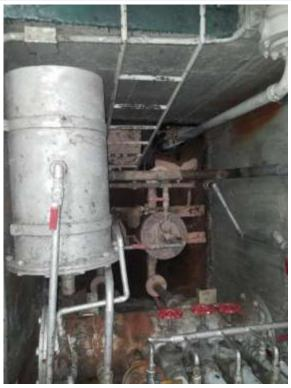
A multiple hazard Confined Space and namely a Biological Purification System pumphouse pit; multiple hazards are also here present like mechanical rotating parts, heights, entrapment structures, biological agents etc. Safety / Environmental Bulletin No. 8 December 2016 Powered by: HMS
