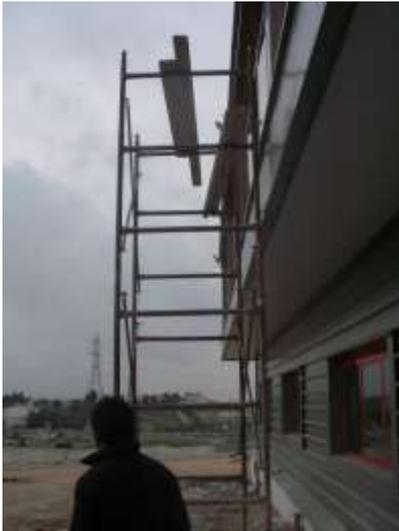
**Maintenance personnel usually use substandard scaffolding especially when the works to be performed are short in duration or of "common nature".**
