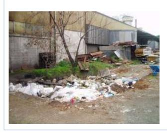
Maintenance debris after a construction work freely dumbed in an open pit for subsequent burning; apart from the direct pollution to the soil, there is perspective pollution to the soil after a rainfall as well as after the uncontrolled waste burning.
