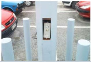
Immediate access to 220V alternative current supply in a parking lot due to poor maintenance (including inspection); note that even a child could be electrocuted since this is a commercial area.
