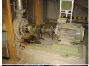
and motor) are misaligned and not properly balanced, more energy is consumed. Energy consumption on the other hand relates directly to many environmental impacts, e.g. global warming, acidification, eutrophication, etc – depending on the energy source. Furthermore, more breakdowns will occur and spare parts will be consumed, which has a direct impact on the environment as well, due to higher material consumption. The noise will level rise.
