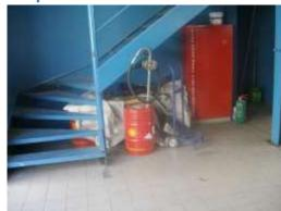
Storage of combustible materials (in this case flammable) under a staircase, not to mention the installation of a Fire Hose as well as other fire-fighting equipment in a semi-accessible area.
