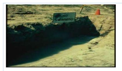
Employees shall not work in excavations where there is accumulated water, or where water is accumulating, unless adequate precautions have been taken, to protect employees (Adapted from the Maryland Fire & Rescue Institute excavation & trenching training module)
