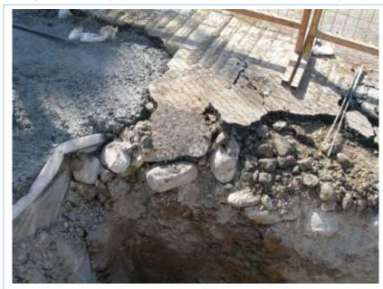
Loose materials should be removed from trenches through a meticulous scaling procedure
