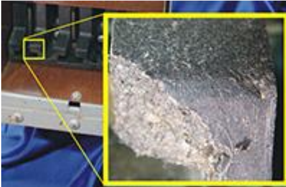
Asbestos was used as insulation in early electrical panels
