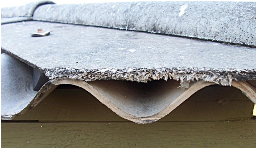
Weathered fibrous asbestos sheeting showing loose fibres
