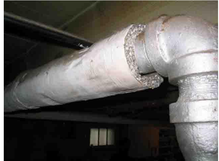
Asbestos steam pipe insulation
