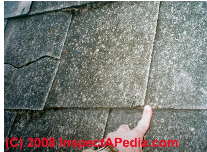
Asbestos in roofing material
