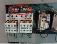
Annual thermal imaging to early detect electrical parts overheating → failure; as one can see visual inspection is not enough
