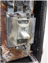
Fire at the Main Power Distribution Panel at a bottling industry; fortunately, the Company had the main Panel Room at a separate area away from the main manufacturing facility.
