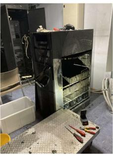
UPS fire incident at a UPS room in a Cinema Complex during the pandemic (November 2020) when the complex was shut down; the smoke detection early warning system went off hence the fire was extinguished by the security guards in time thus preventing the fire from spreading.
